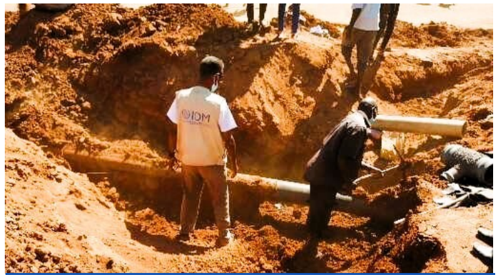
Rehabilitation of the local water network to ensure access to safe water for communities in Kassala state amidst influx of IDPs. © IOM SUDAN 2024
