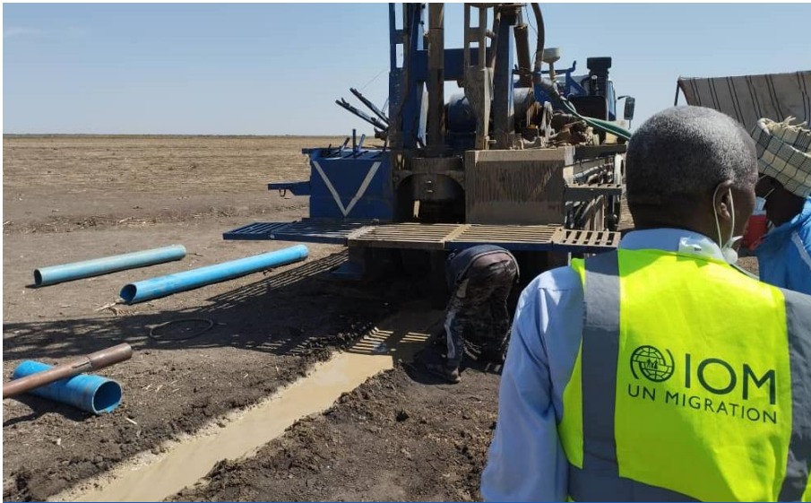
Drilling of borehole in Sennar state. © IOM SUDAN 2024
