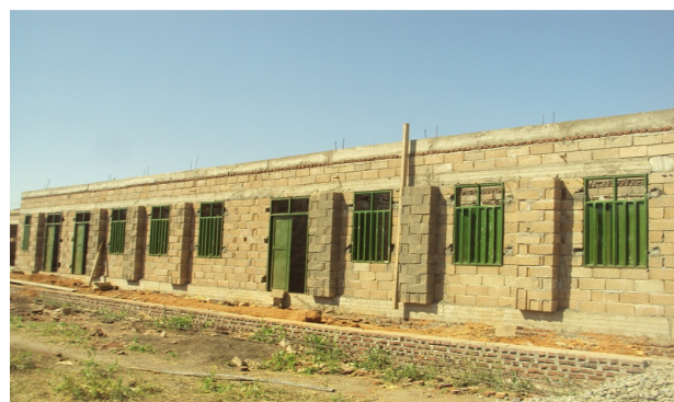
Figure 4: Primary school under construction, Blue Nile
